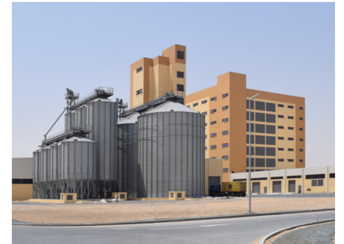
↑ Compound feed plant: throughput capacity up to 245 000 t/a
